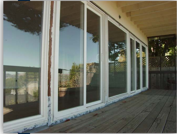
Partial Window Replacement
