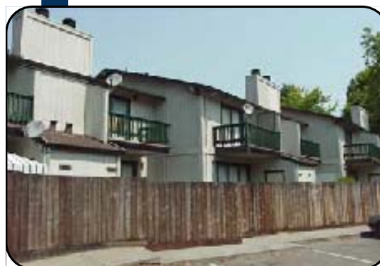
Back Side View of Units
